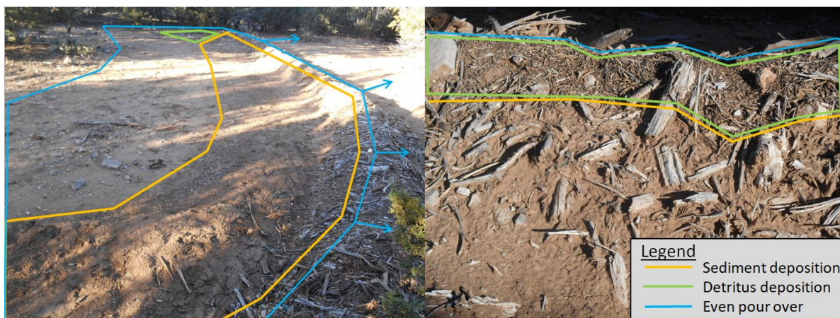
Figure 15: A wood chip berm built by Christian Meuli in NM harvests water, sediment, and organic detritus during a monsoon rain event. Water is retained for infiltration and eventual sheet overflow across the level top of berm (left). A close-up view of the wood chip berm shows sediments embedding the wood chips (right). Sediment-detritus line mirrors the high water mark and shows the relatively even spill over.
