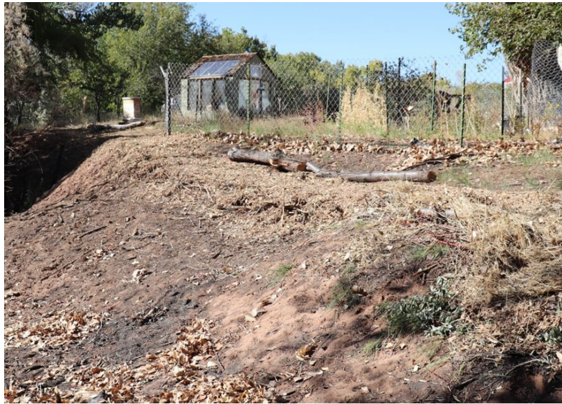
Figure 3: Woody materials from a fire damaged landscape are laid across the slope and covered with a soil-wood chip mix creating a path that harvests runoff and stops erosion.
