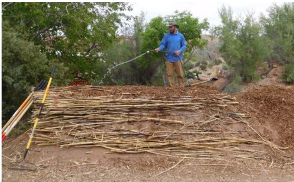
Figure 39: Watering your structure can increase decomposition and promote vegetation establishment
