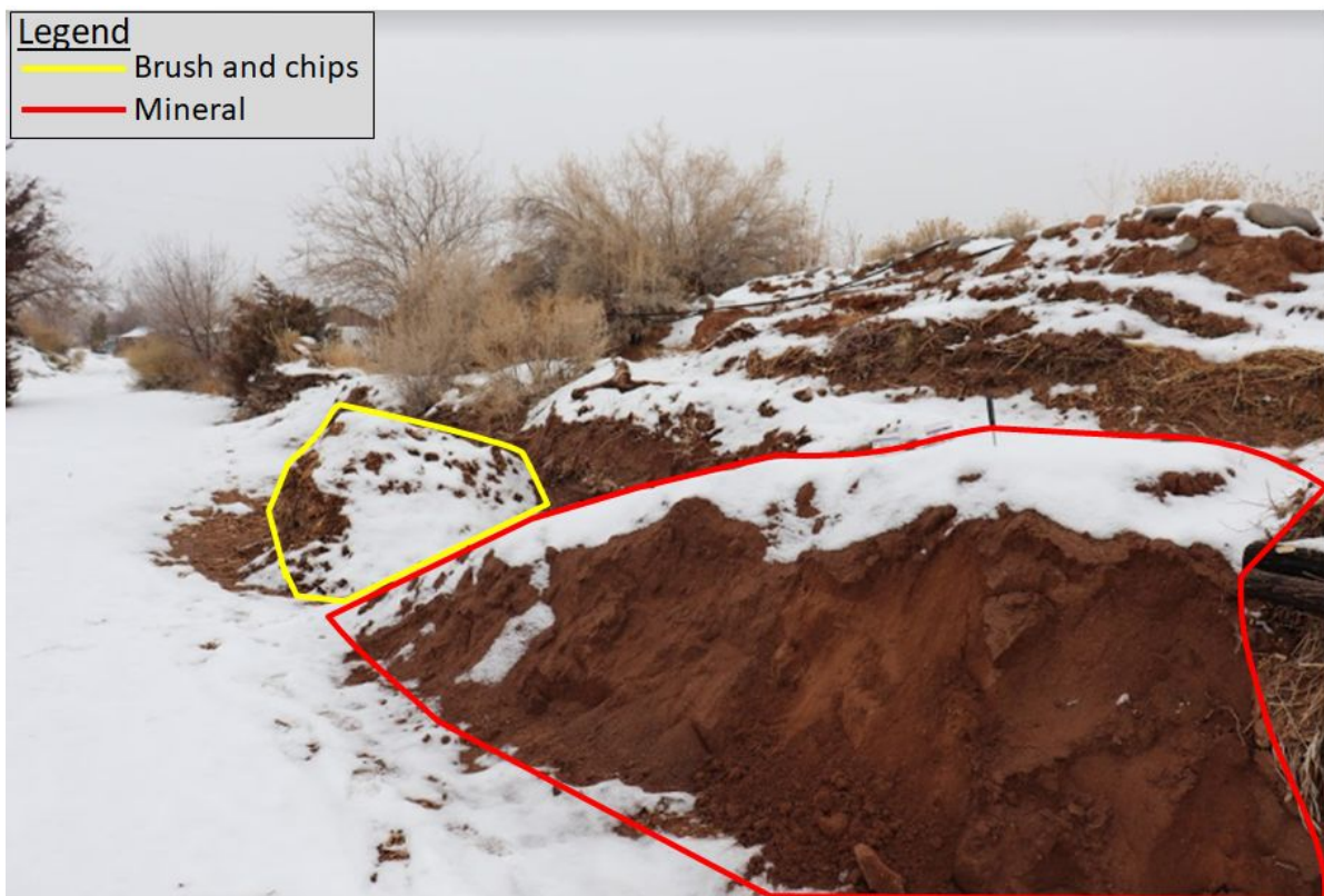
Figure 28: Bulk piles of purchased mineral and wood chips are staged for easy access by wheelbarrow or truck. Access is kept open for other deliveries and site activities
