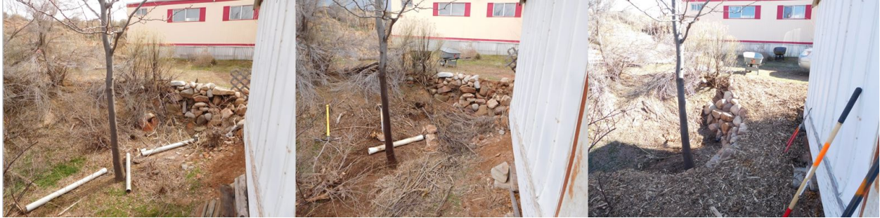
Figure 7: A rock wall made access to part of the property difficult (left). Densely layered brush and soil (center) are used to create a ramp that provides easy access to this area of the property (right).
