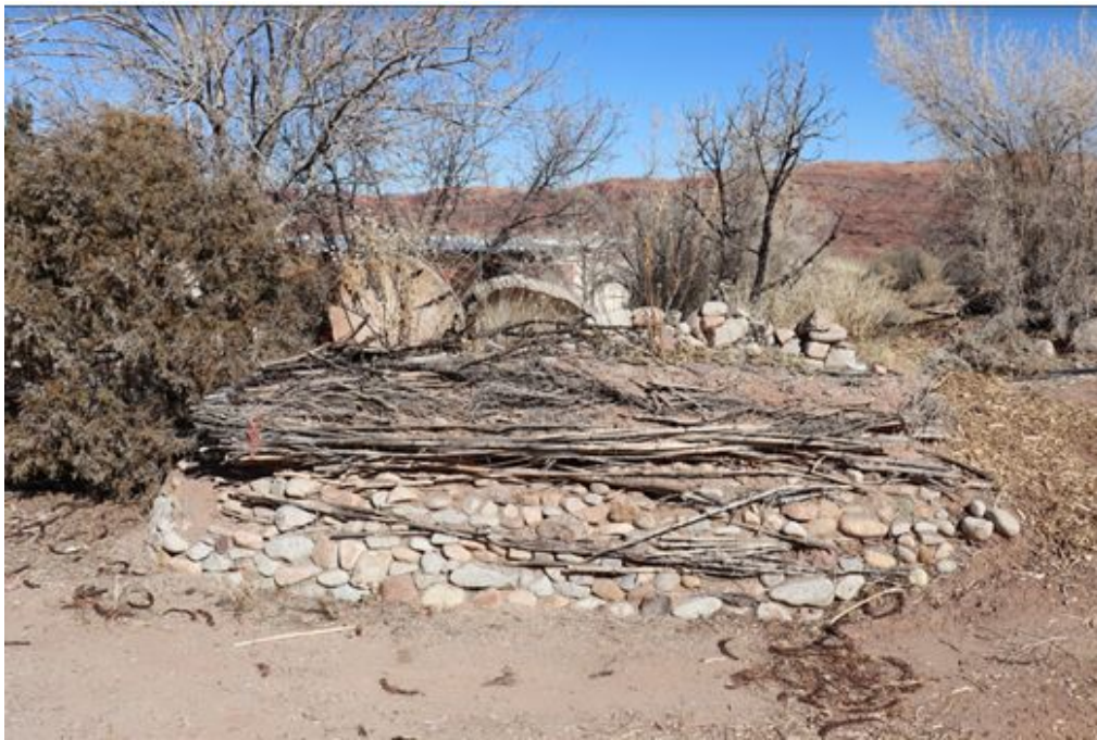
Figure 41: Structures can continue to evolve over time, like the log rounds and rocks used to increase the height of this berm and provide a suitable micro-climate for plant growth.
